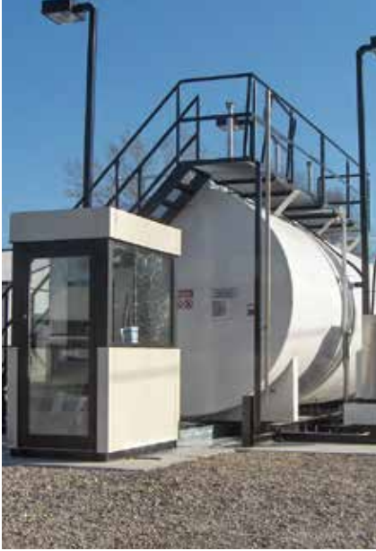
OPW-RF AST installation
