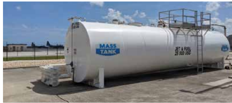
Above ground UL 142 Flameshield tank
